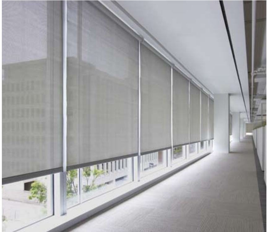
As seen here at the U.S. Green Building Council headquarters in Washington, D.C., in uniform mode, the shades can only be moved to one of five factory-preset or user-defined positions.
