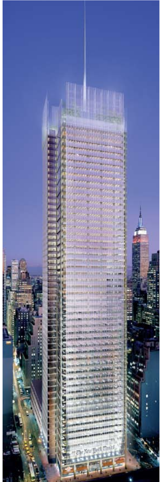
The SolarTrac® System has been implemented in The New York Times Headquarters.
